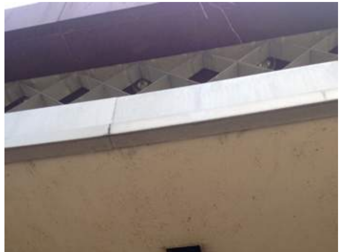
A12 _Replace Mt. Pleasant Ave. entrance area soffits and lighting
