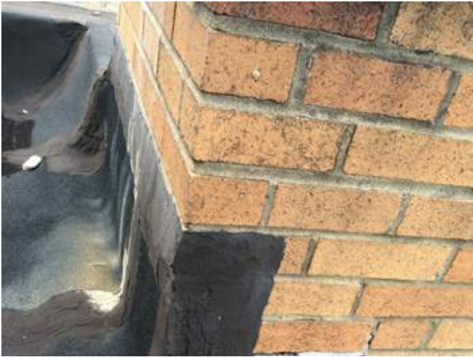
A7 _Chimney cap stone replacement and flashing
