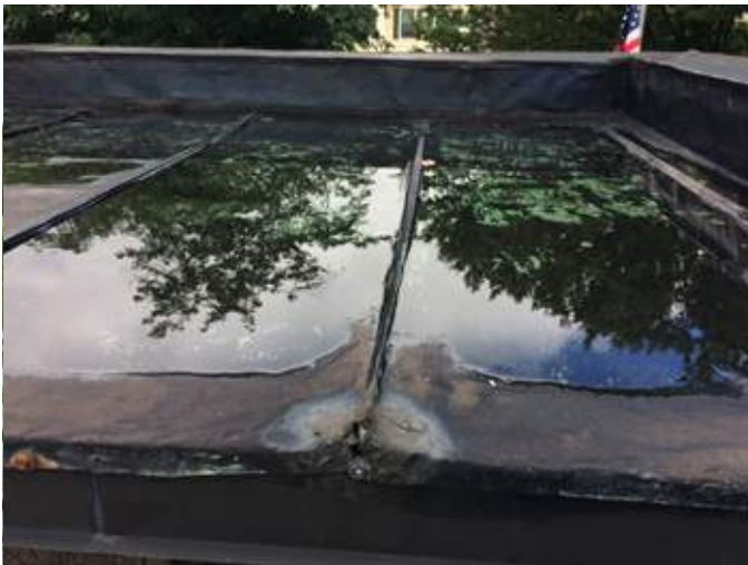
A3 _Roof replacement and new coping at original building
