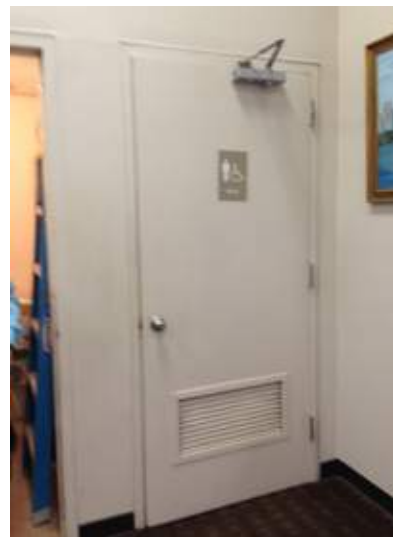
A28 _Modify public restrooms for ADA compliance
