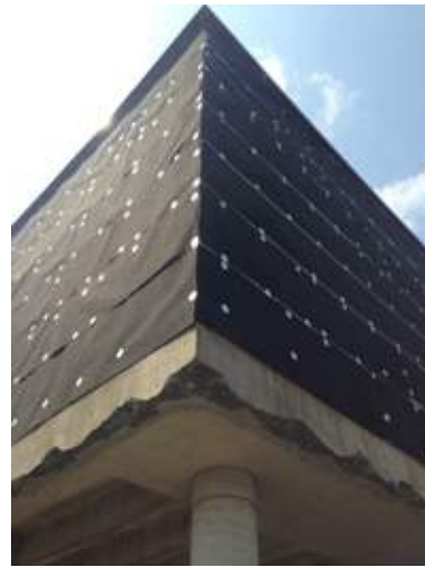
A2 _Brick facade replacement at 1978 addition
