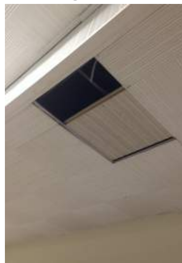
A24_Replace ceiling at lower level storage/stack area
