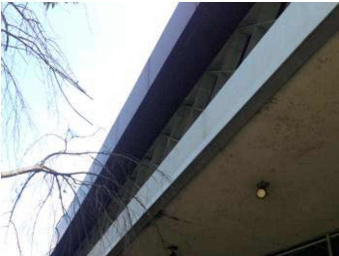
A11 _Replace Mt. Pleasant Ave. entrance area soffits and lighting
