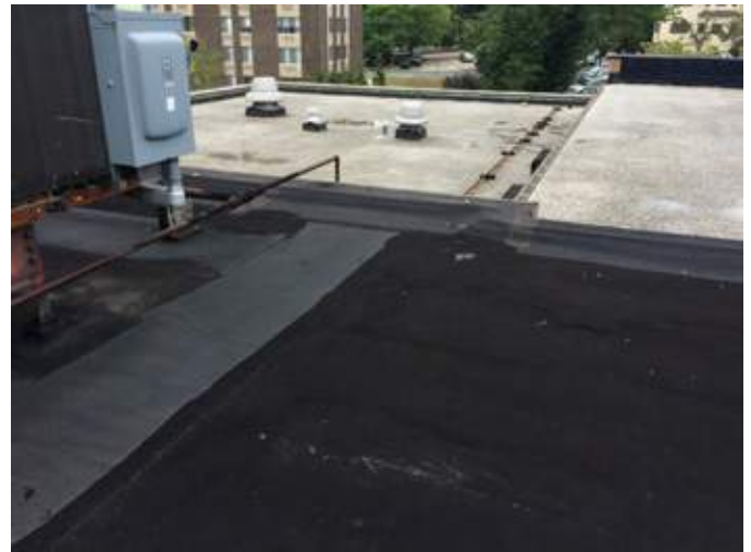
A4 _Roof replacement and new coping at original building
