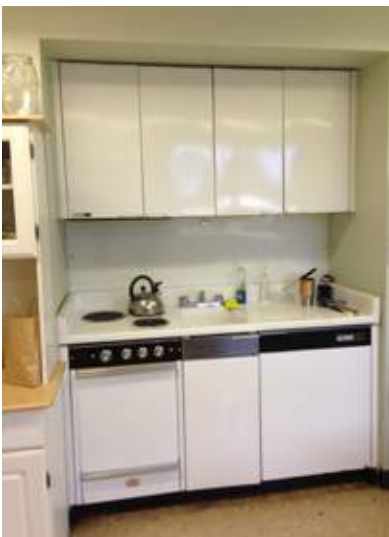
A27 _New kitchen counter, sink and appliances
