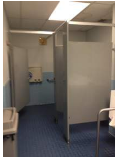
A30 _Modify public restrooms for ADA compliance
