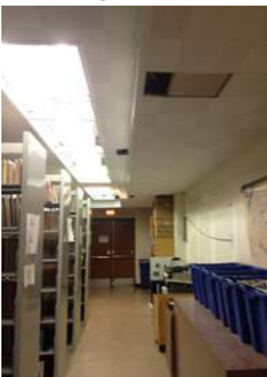
A23_Replace ceiling at lower level storage/stack area
