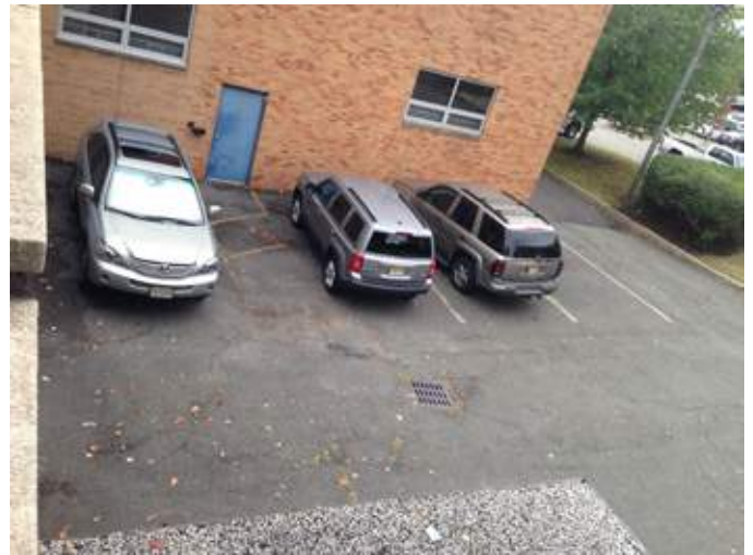
A10 _Exterior hollow metal door painting
